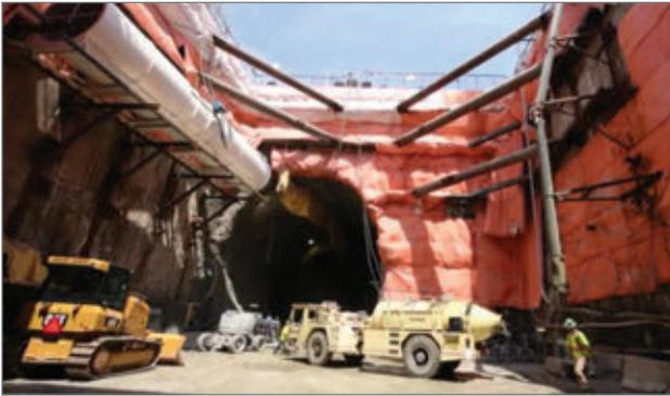
Figure B – Large area excavated for an underground LRT station<sup>2</sup>
